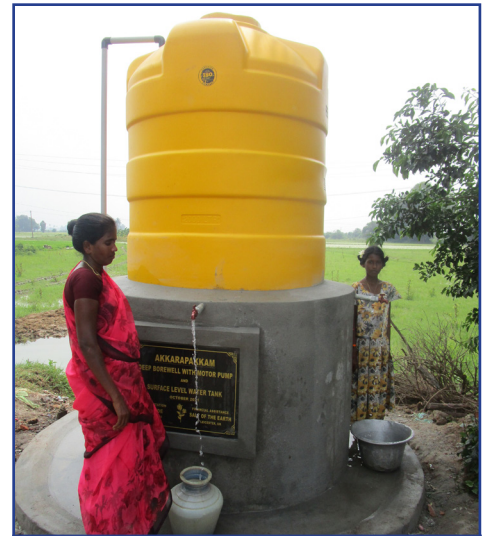
Akkarapakkam pump in use
