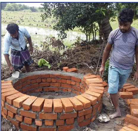
Akkarapakkam pump construction
